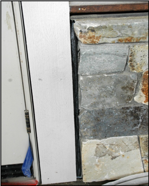
Prepare Joint with Backer Rod
