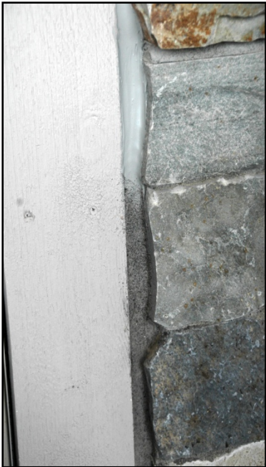
Apply Sand into Sealant
