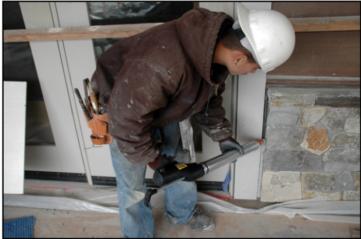
Delivering Sealant to the Joint Cavity
