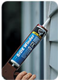
Sealant applied to siding. Photo courtesy of DAP.
