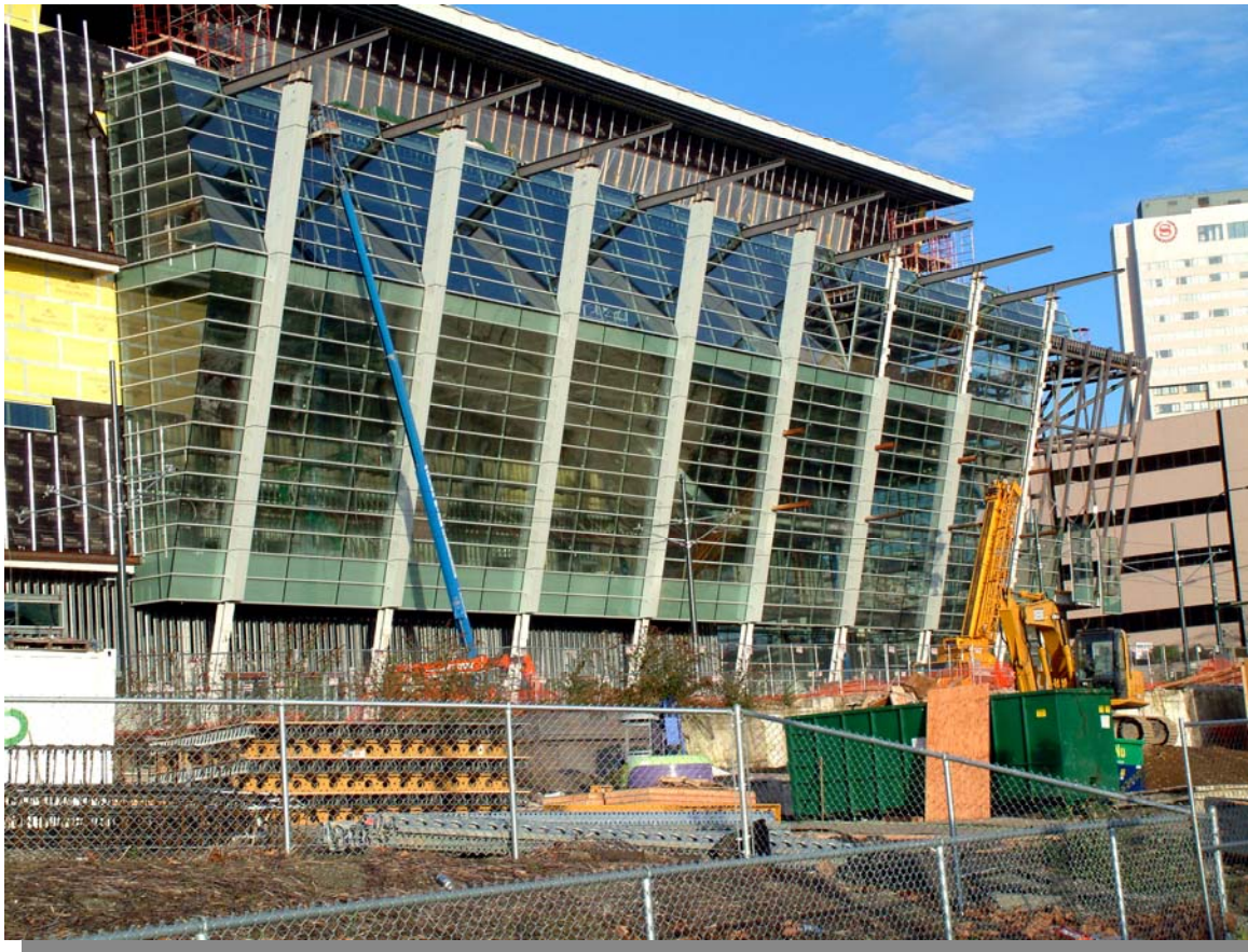
Non-porous surfaces of glass and glazing
