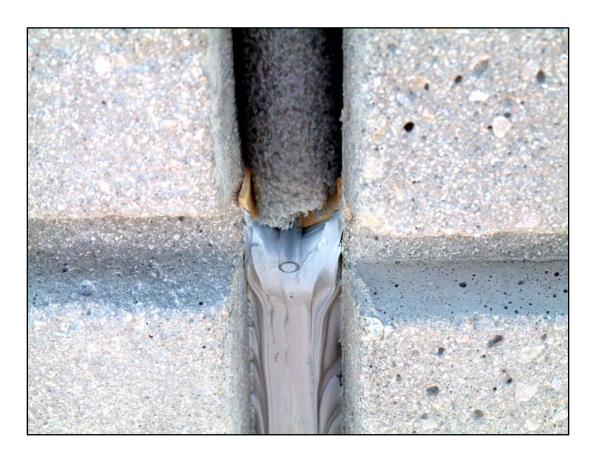
The weep tube is placed before the final sealant bead is installed.
